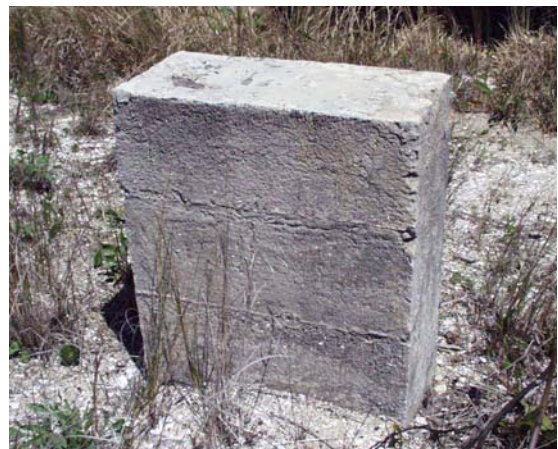
Figure 20 View of typical concrete pier. (NPS-SERO-CR, 2002)
