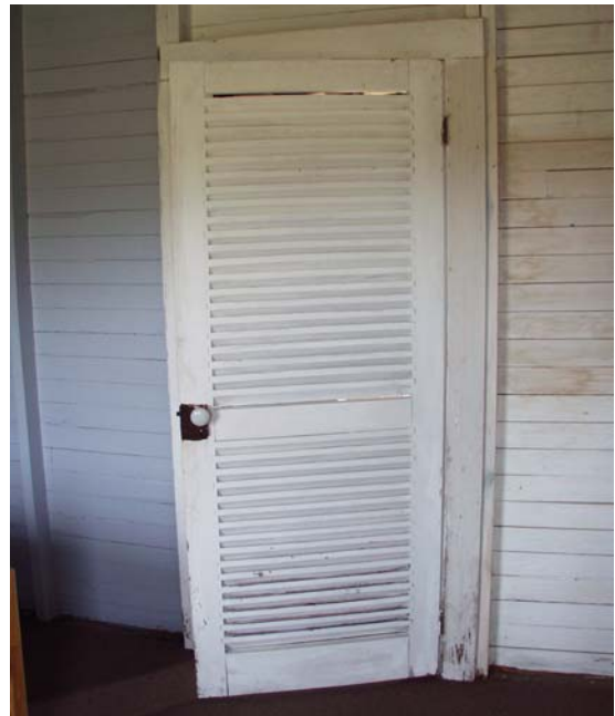
Figure 27 Typical bedroom door with rimlock and porcelain knobs. (NPS-SERO-CR, 2003)
