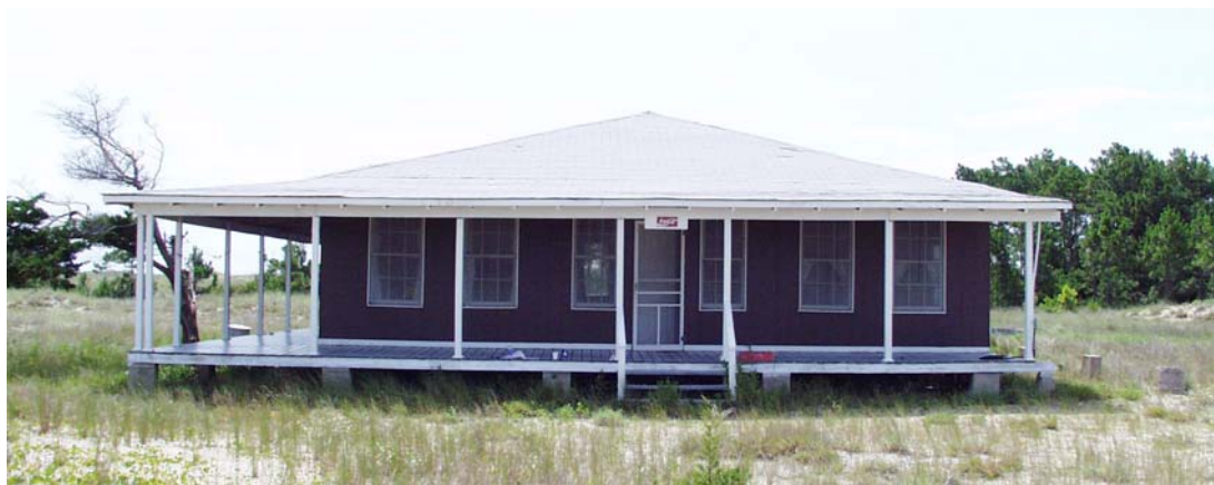
Figure 16 View of front (northwest side) of Coca-Cola House. (NPS-SERO-CRS, 2002)
