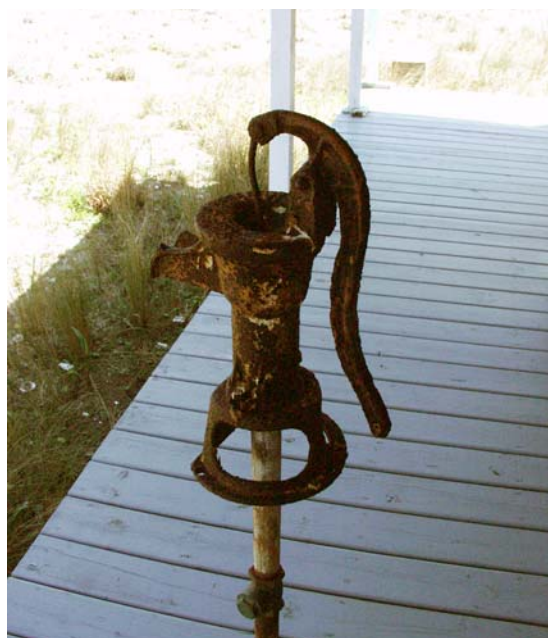
Figure 34 Hand-operated water pump on northeast porch. (NPS-SERO-CR, 2003)
